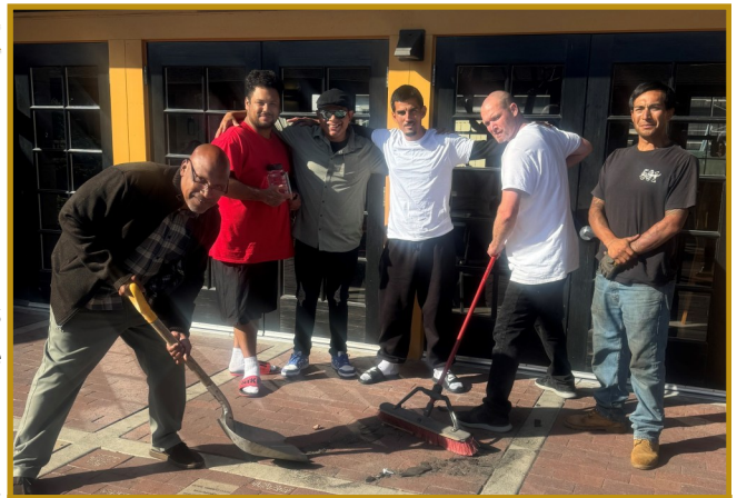
Men's Residential during roof installation at the Andy Church Hall and Fellowship Hall.
